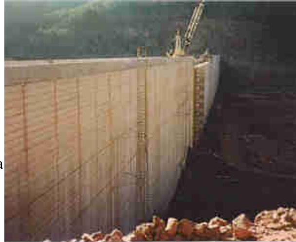
Figure 1. The Stillwater dam in Colorado used roller compacted concrete (RCC) which has properties similar to Roman concrete.
